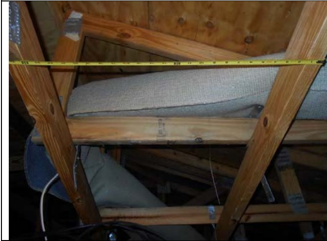
TRUSS SPACING 24"
