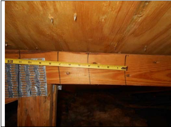
FASTENER SPACING
