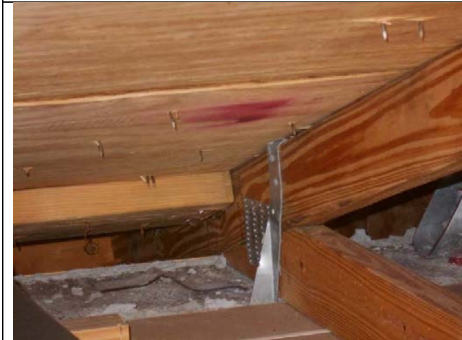
WALL CONNECTION - STRAPS ROOF TO WALL CONNECTIONS.
