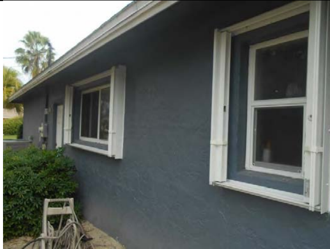
WALL CONSTRUCTION TYPE - CBS
