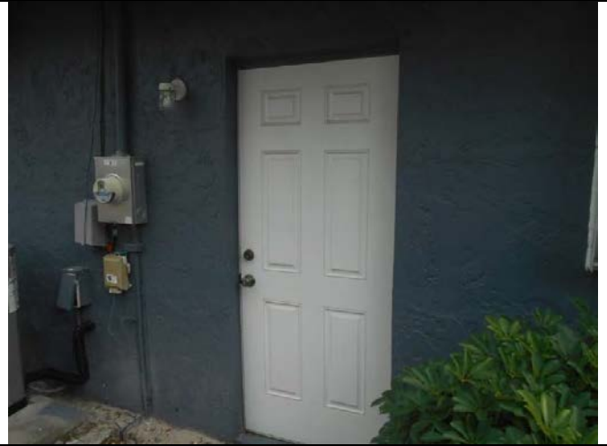
ENTRY DOOR – PROTECTED
