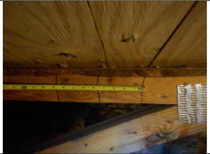
FASTENER SPACING
