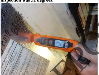
Temperature difference was not within the 16 to 22 degrees normal operating range at time of inspection. Suggest review by a qualified HVAC contractor.
