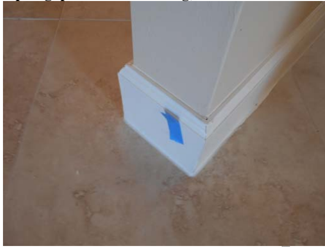
Improperly finished doors and trim;
