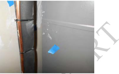
1806.FilterReview; Located at the unit. Home was not even broom clean at<br/>the time of inspection and construction dust/debris not<br/>protected from return air locations. Ductwork should be cleaned<br/>and filter replaced after final cleaning completed.
