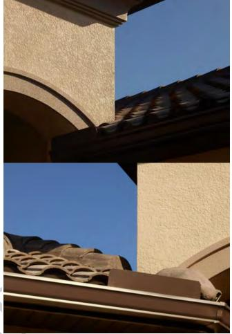
**Review;** Cleaning of all roof tile required. Paint over spray and construction debris noted.
