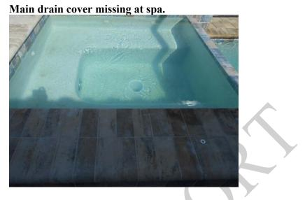
Spa emptied when put in spa function and pool overflowed; pool not properly set up and not all equipment installed properly. Pool installation incomplete.
