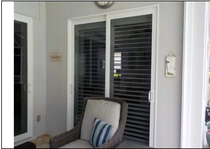
ENTRY DOORS – PROTECTED
