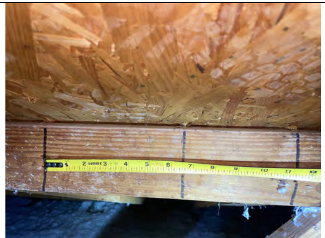
FASTENER SPACING
