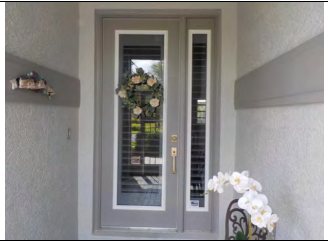
ENTRY DOOR – PROTECTED
