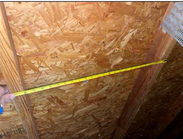
TRUSS SPACING 24"
